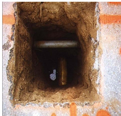
Fig 2.4 Utilities in a Test Hole
