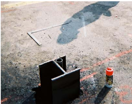
Fig 4.1 Pile Driven within 1’ of Utility
